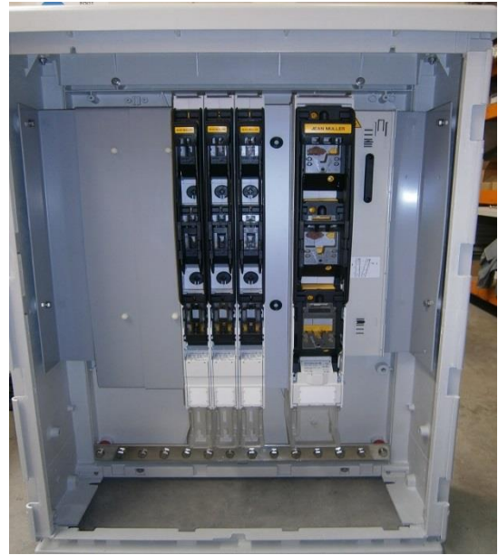
NKVS1 6-way with N/E bar
