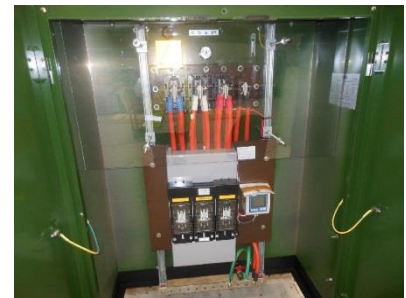
LTLA-3X3/9/1250 & 1600 configurations with & without MDI up to 1MVA.
