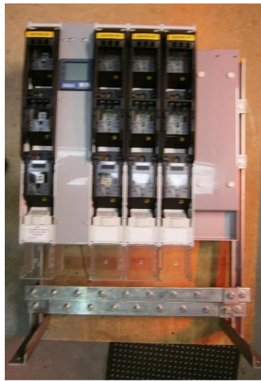
7 way Free standing LV rack with internal MDI, 2 spare 100mm ways & N + E + link bus bars.
